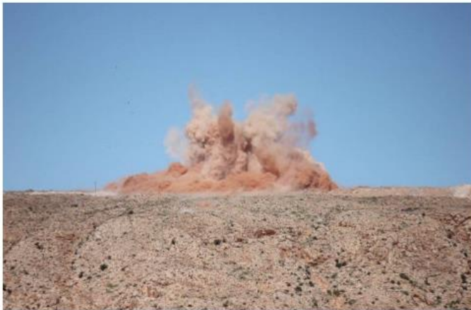
The first blast at Vedanta's Gamsberg mine
